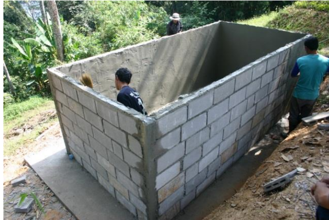
Figure 2 Concrete water storage
