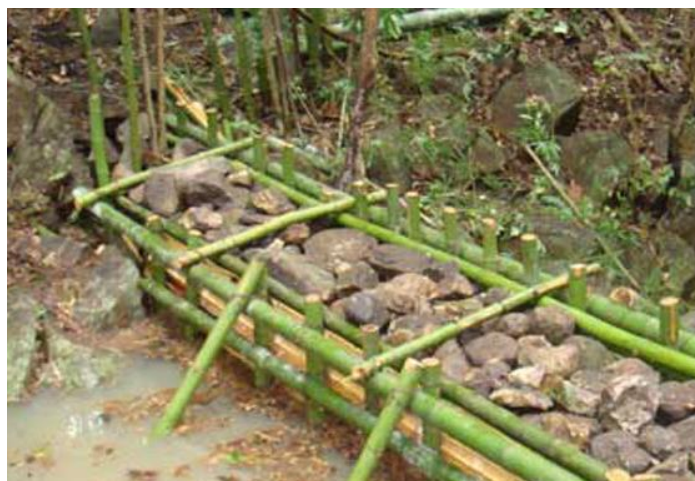
Figure 3 Rock-bamboo check dam
