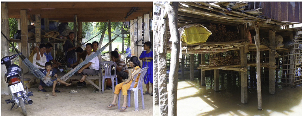
Figure 3. Elevating the house floor as part of flood mitigation measures in rural areas of Vietnam (Liao et al. 2016)
