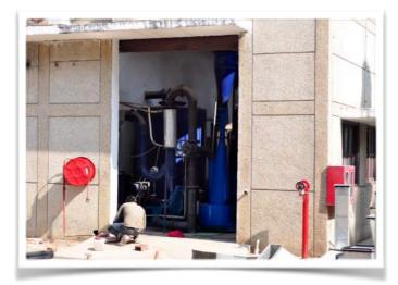
During visited to Biomass gasifier plant, the technical person explained the process of the system. The process started with **burnt twice as efficiently the wood waste, branches, twigs, firewood and crop stubble** inside the reactor. Energy that generated is used to power the TERI's building by connecting with the smart mini grid as a centralize energy distribution.
