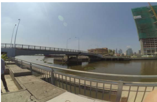
Fig. 3 Flood Prevention Gate
