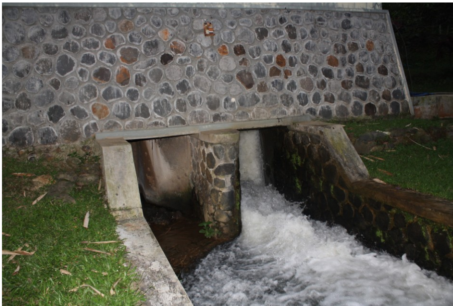
Figure 1: Dam, Diversion Weir and Intake
